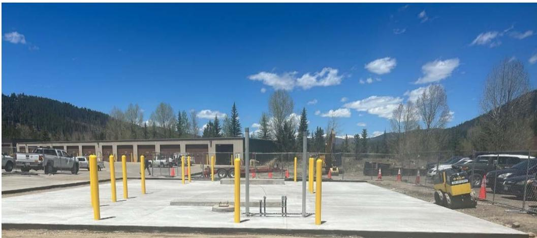
Concrete has been poured for the fuel island.
